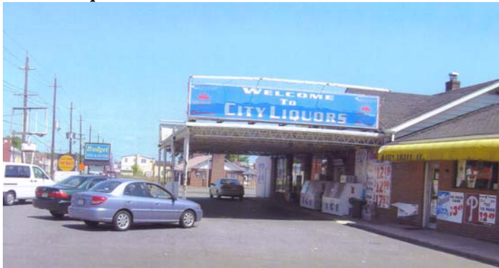
Canal's Liquor Pre-Construction
