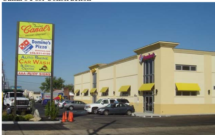
Canal's Post Construction
